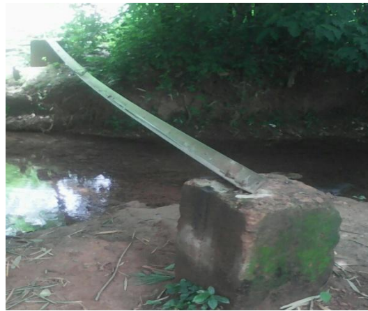
Plate9. Narrow Iron Bridge, a tourism facility in Ezeagu tourist complex
