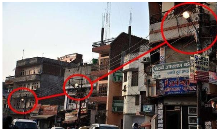
Fig2. Improper Monitoring of Street Lights
