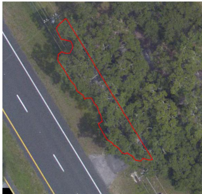
Figure22. Vegetation inside a polygon obstructs the power line.
