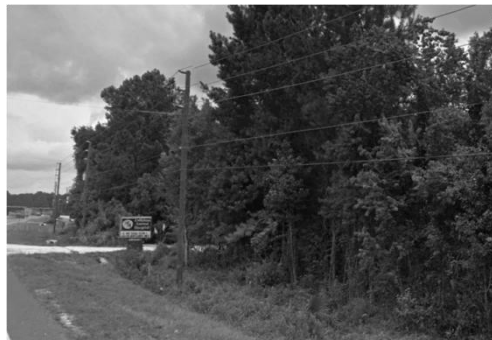
Figure4. Power lines in the study area
