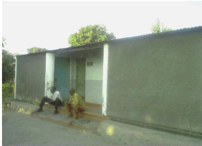
Plate9.7: Showing a partially improved low-cost house with the owner and son seated
