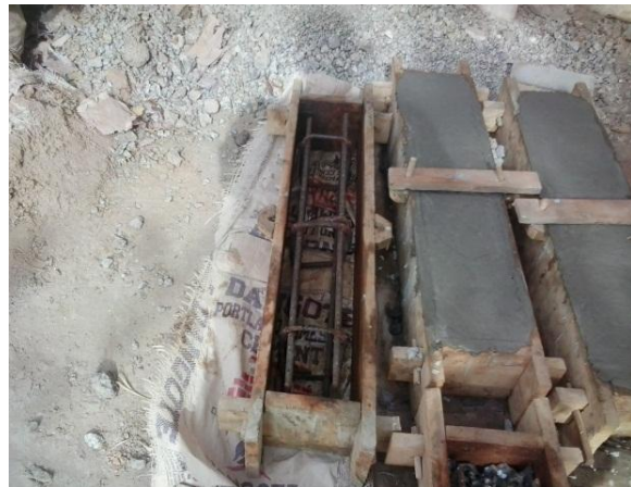
Plate II. Casting of concrete Beams
