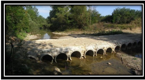
Vented Causeway at Feccia River(Italy)
