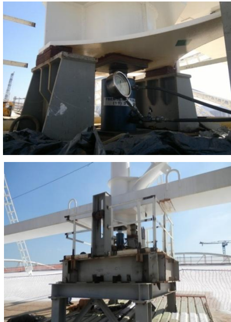
Figure11. Shimming, hydraulic devices and lateral guides installed(João Havelange Stadium, Rio de Janeiro, Brazil).
