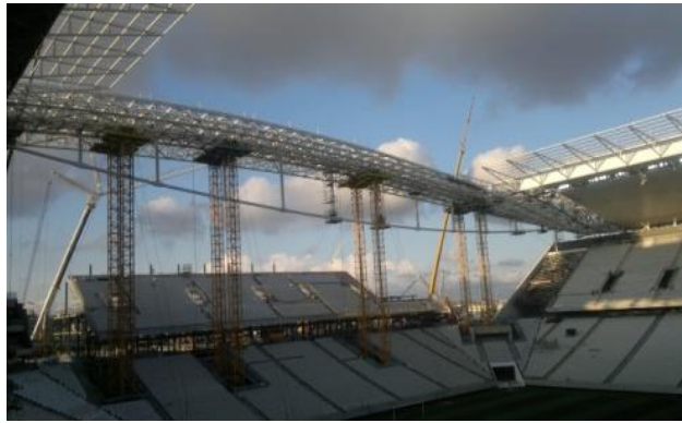
Figure1. Erection of the roof of the Corinthians Arena, in São Paulo, Brazil
