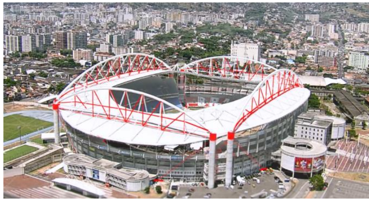
Figure20. An overview of the reinforcements installed on the roof structure of the João Havelange stadium.
