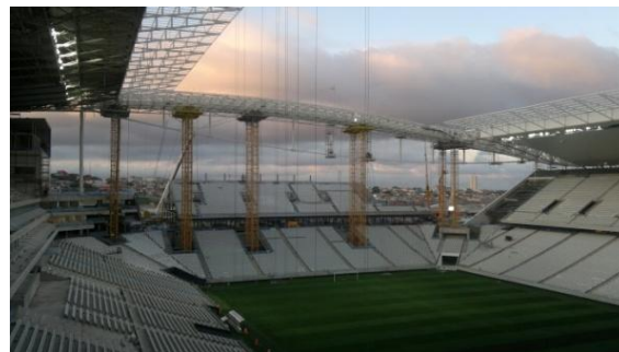
Figure16. Northern Truss of the Corinthians Arena during the erection phase.
