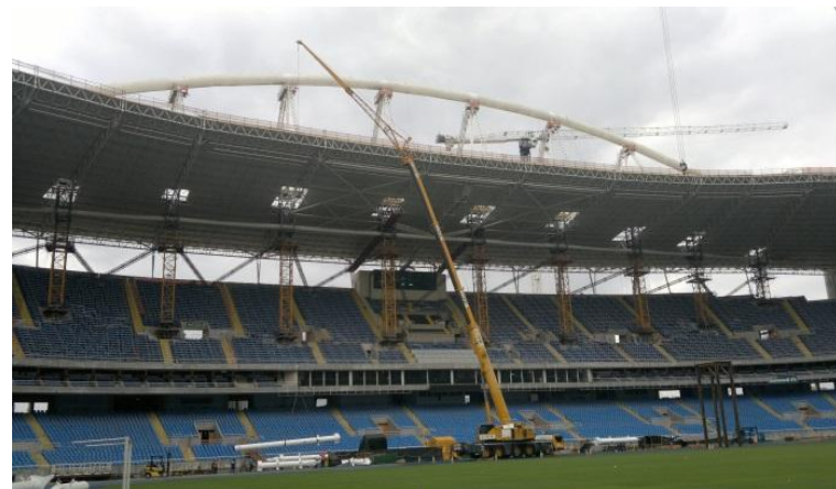
Figure21. Temporary towers to support the roof prior to the installation of the reinforcement.
