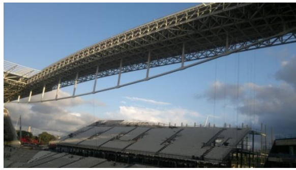
Figure15. Southern Truss of the Corinthians Arena, erection stage just finished.
