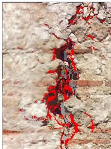
**Fig. 7.** Detail from main façade. Isolated point cloud, the colored red points (8412 out of 42809) highlight the basic outlines of this wall part pathology. Lack of monuments material.
