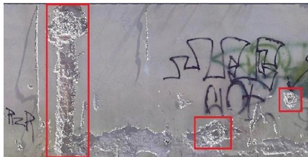
**Fig. 4.** Orthoimage of southeast façade. White spots highlight the outline of the pathology detected. The chosen combination of the parameters k and coef is 21 and 1 respectively.
